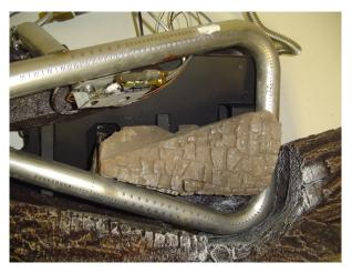
Figure 20A - Installing Charred Log Top View
